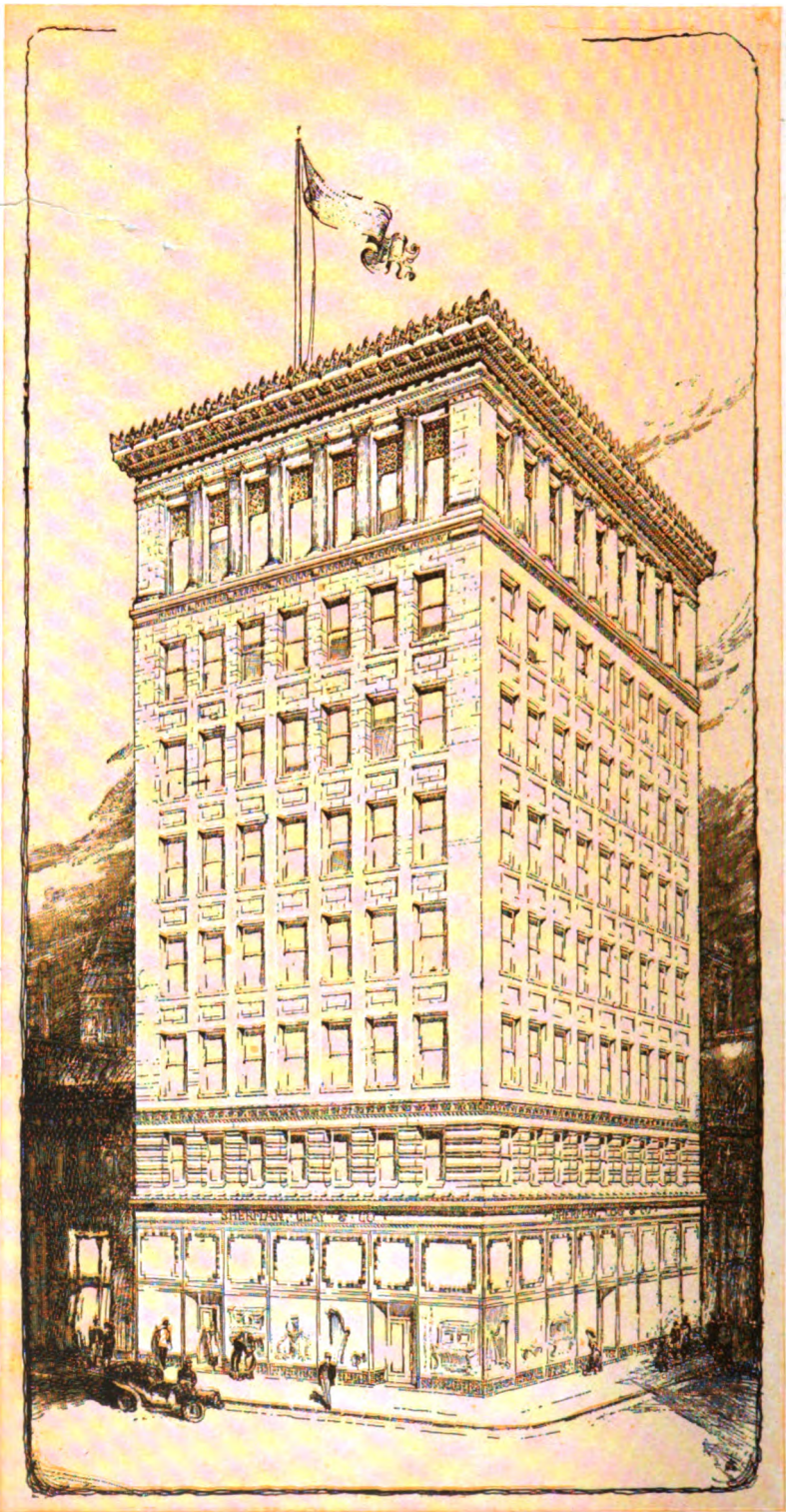
THE NEW HOME OF SHERMAN, CLAY AND COMPANY, MUSIC DEALERS, SOUTHWEST CORNER OF KEARNY AND SUTTER STREETS; COST, ABOUT $220,000; A STEEL FRAME BUILDING FACED WITH GLAZED TERRA COTTA; ARCHITECT, L. B. DUTTON
